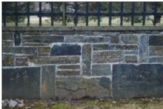
Appropriate: Mortared stone wall
