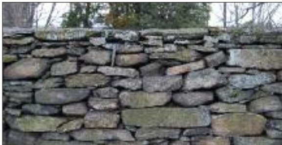
Appropriate: Dry stacked stone wall
