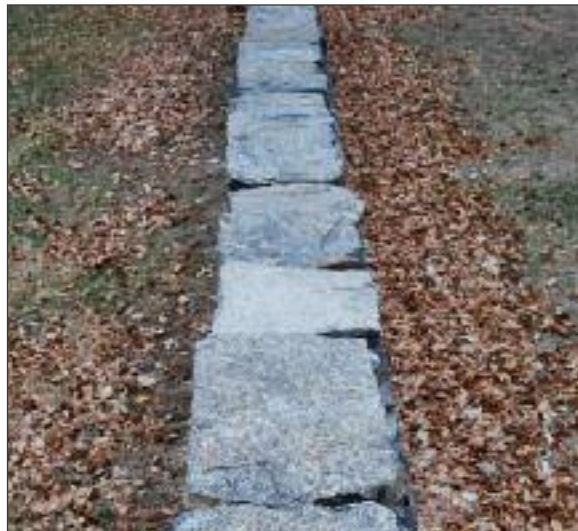
Appropriate: Cap on dry stacked stone wall
